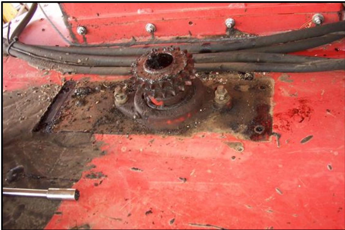
Fig. 6-5 Removal of Motor Mount Assembly
